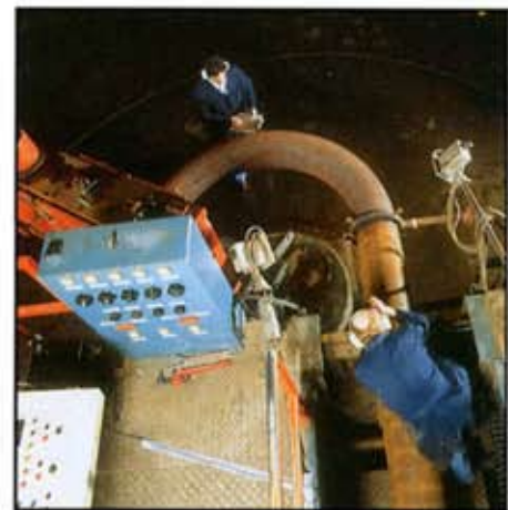
Q.A. technician monitoring wall thickness with ultrasonic equipment.
